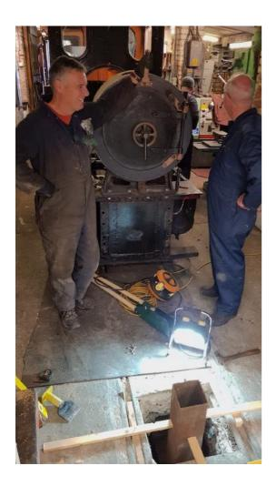
A big hole has appeared in the Engine Shed! Not a sinkhole caused by recent deluges but an excavation for a new buffer stop, just beyond the new party room. The stop will be removable, sliding up and down in a sleeve concreted into the hole. That way the doorway access can be kept clear.
